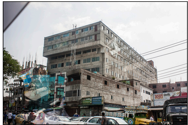
"Photo of Rana Plaza taken one year before the collapse" by Sean Robertson is licensed under CC BY-SA 4.0.
